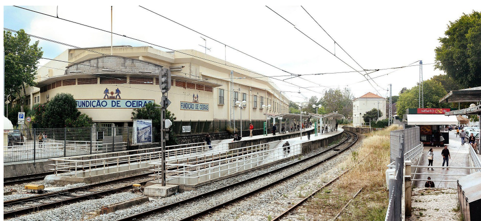
OEIRAS TRAIN STATION
